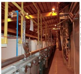
The system is designed for personnel to carry out superior vacuum cleaning duties from specific pieces of production equipment and surrounding area.
