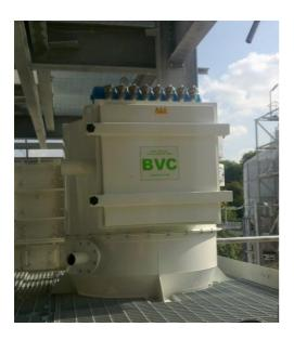
The motive air is generated by an exhauster unit powered by an 18.5 kW motor. The unit is located on an automatic self-tensioning drive system, within a force draft ventilated acoustic enclosure with discharge silencer ensuring low noise levels.
