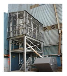
Motive conveying air is generated by a positive displacement exhauster powered by an 18.5 kW motor, fitted in a force draft acoustic enclosure, reducing the noise level down to below 70 dB (A) at 1 metre free field.
