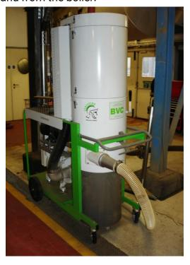
There are 12 hose connection points installed through 6 floor levels, with interconnecting pipe work back to a BVC static industrial vacuum cleaner.
