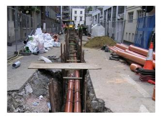
theory, the challenge was to physically run 4 x 160mm tubes along the interconnecting route, much of which would require installation underground.
