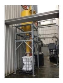
Motive conveying air is generated by a positive displacement exhauster package powdered by a 15.0 kw motor provided with all necessary ancillaries and located within a force draft ventilated acoustic enclosure ensuring noise emission level is kept below 75 dB(A) at 1 metre measured under free field conditions.
